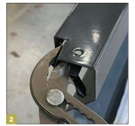
Use a pair of pliers to rotate and twist the tab. TO BE done before mounting the plate between the posts.
