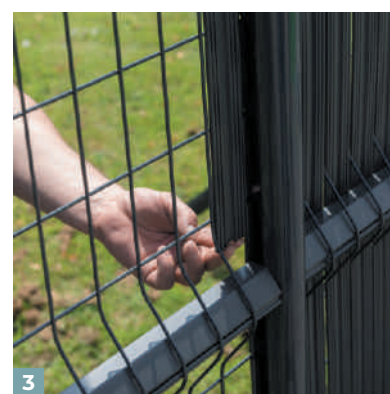
3 Identify the 2 end slats (45mm). Slide them in the first mesh at each end of the panel, with the tab facing the fold .
