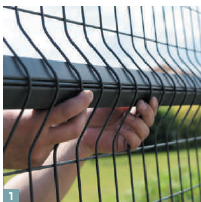
1 Position a reinforcement element in the first fold of the panel (top).
