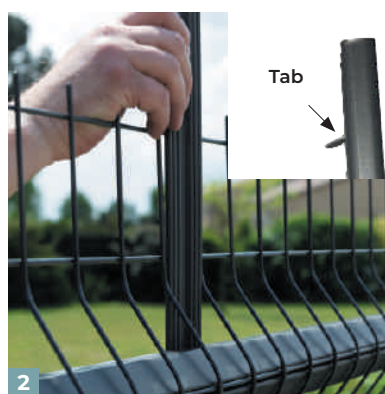
2 Slide a slat (48mm), with the tab facing the fold , into a mesh in the centre of the panel to maintain the reinforcement element. Slide it up to the next folds. Repeat the operation for each of the folds.
